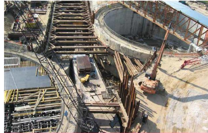
Temporary Works for Shafts and Pipelines
