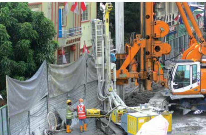
Rock Fissure Grouting
