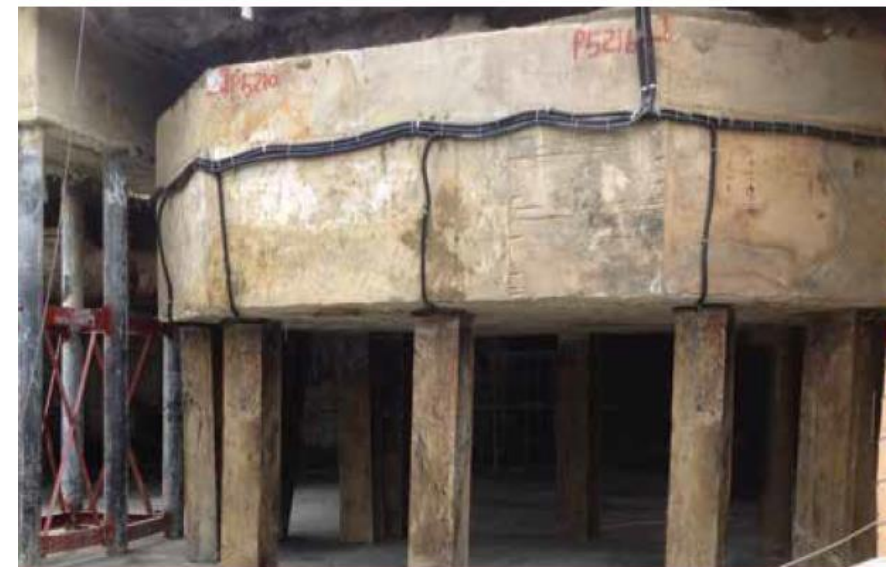
LRT Viaduct Pier P521 Underpinning
