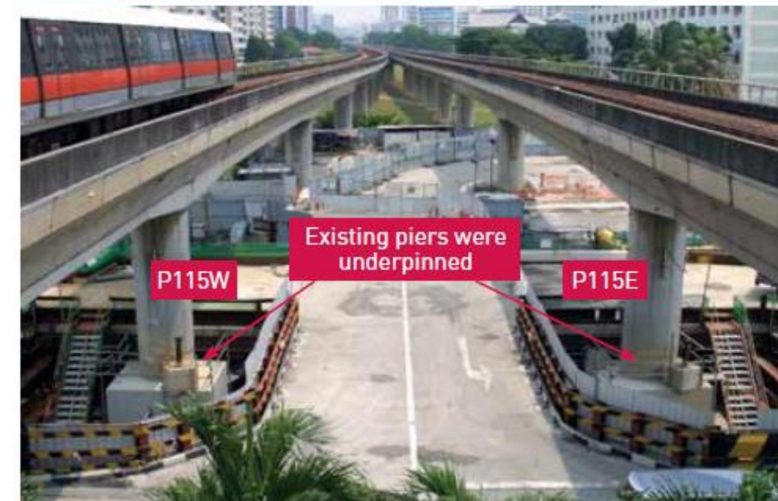
Photos of Existing Piers that Require Underpinning
