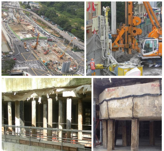
Clockwise from top left: Traffic Diversions at Project Site; Rock Fissure Grouting; LRT Viaduct Pier P521 Underpinning; Canal Underpinning
