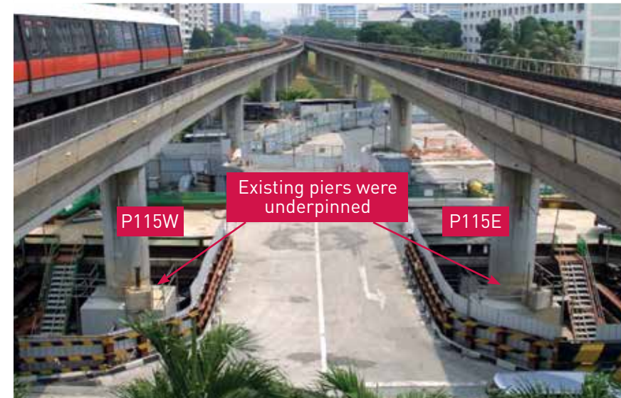
Photos of Existing Piers that Require Underpinning
