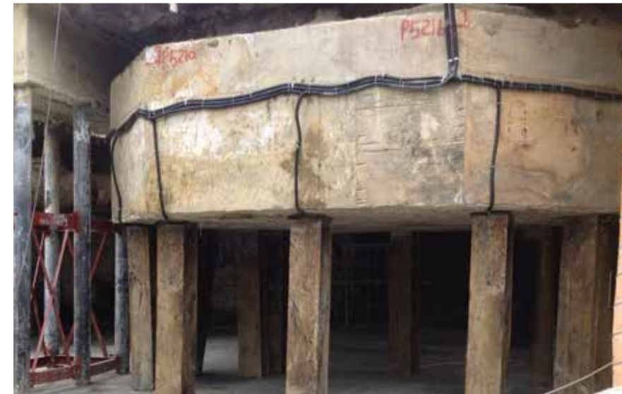
LRT Viaduct Pier P521 Underpinning
